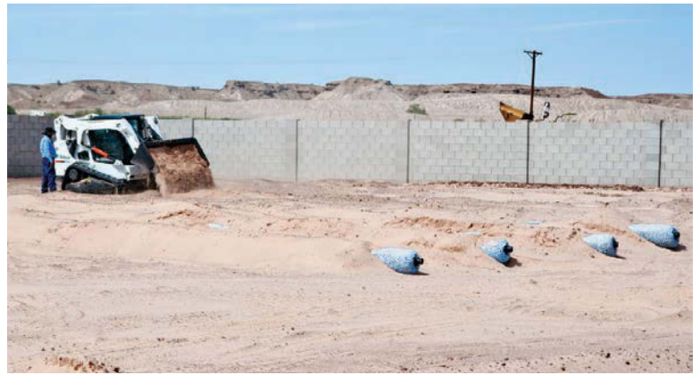
Workers from Westar Plumbing Services in Yuma, Ariz., distribute sand to form an evaporative bed for the wastewater system at J & A RV Park in Winterhaven, Calif.
