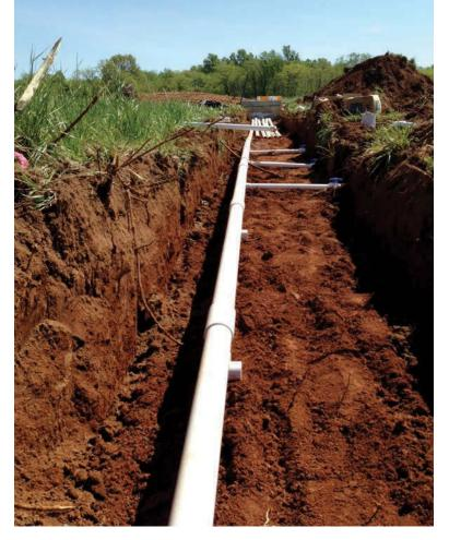
Laterals within each zone were laid 5 feet on center, and the spacing between zones varied from 5 to about 30 feet. Approximately 16 to 18 inches of native topsoil covered the laterals.
