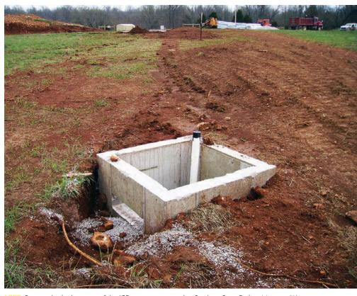
**LEFT:** Pipe marks the locations of the LPP zones constructed at Stockton State Park in Missouri. Wastewater is dispersed in a total of 12 zones, each about 150 feet wide and 300 feet long. **ABOVE:** This concrete box holds a six-position indexing valve to distribute wastewater among the LPP zones. The valves were buried above the frost line and drain when they are not active.
