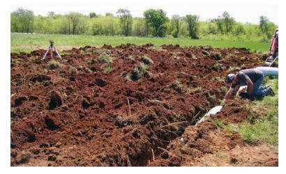
**ABOVE:** A member of the Travis Hodge Hauling crew checks a trench during installation of EZflow from Infiltrator Systems at Stockton State Park. Laterals were above the frost line, but that kept the crew from digging through the tough Missouri hardpan.
