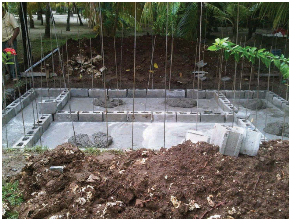
The base for the treatment tank is laid out on Anthony's Key. Because of the expense and difficulty of getting any sort of finished building material to Roatan, most structures are built of concrete, cement and sand, which are shipped in bulk. Tanks like this are constructed from cement blocks molded on Roatan.
