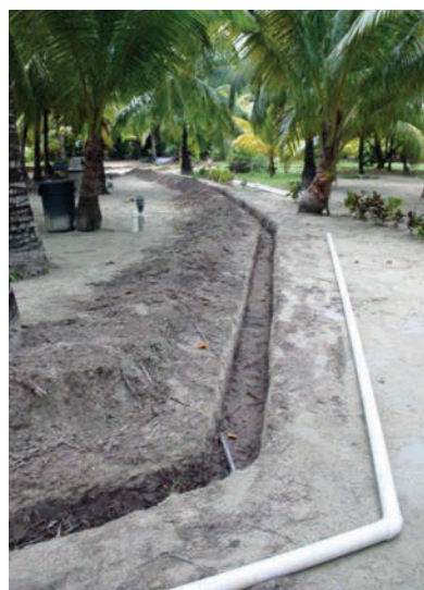
Gravity sewer taking wastewater from divers' cabins to collection tanks had to be routed around the palm trees that dot Anthony's Key. Below the sand, sometimes only a couple of inches, is old coral so hard it will break jackhammer bits.
