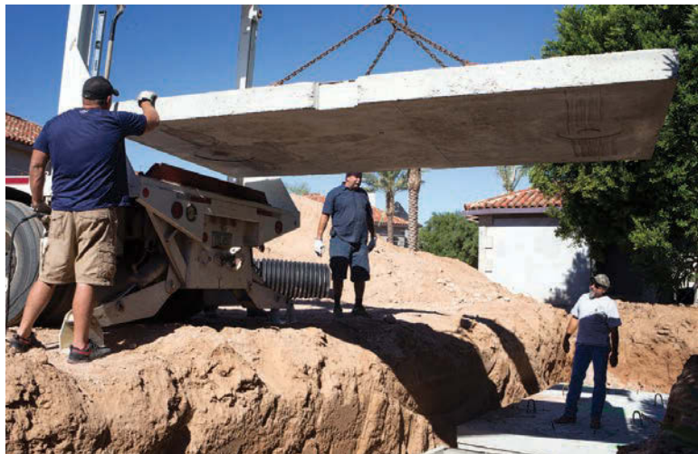
ABOVE LEFT: Tim Bottorff, at the controls of a Cat backhoe, installs a 10,000-gallon water retention system for a Paradise Valley home.
