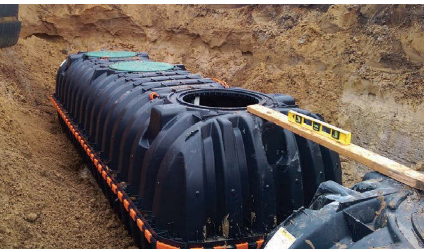
A pair of 1,500-gallon Infiltrator IM-1530 tanks serve as equalization and dosing tanks for the Eljen sand filter installed at an assisted living facility in Auburn, Michigan.
