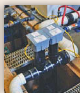
Nursing Home, OH 2 Salcor 3G UV Units in Series with an Activated Sludge Plant. Replaces Chlorination
