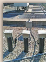
Elementary School, MO 3 Salcor 3G UV Units in a Parallel Array
