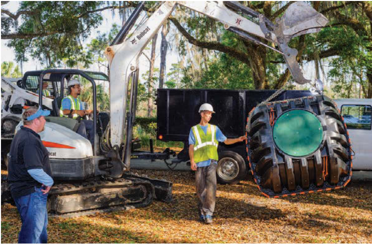
ABOVE: Gaston Montes uses a Bobcat mini-excavator to move an Infiltrator IM-540 tank into place during an onsite system installation. Technician Cody Cummins guides the tank, while Southern Water and Soil owner Greg Mayfield, left, looks on.
