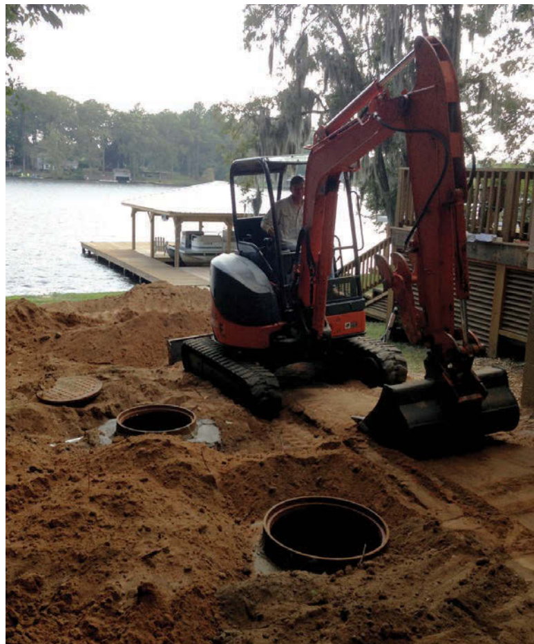
Workers use a Zaxis 35U mini excavator from Hitachi to finish installation of the new treatment tank. Effluent from the tank is pumped uphill to the drainfield.
