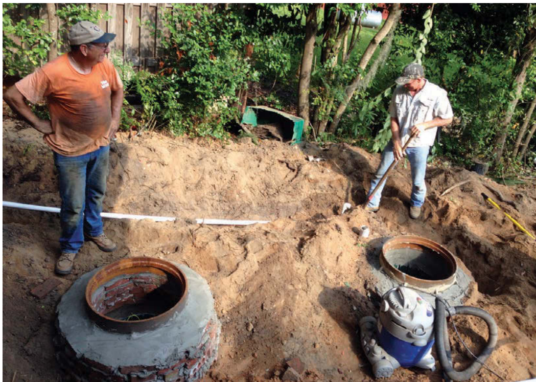
Workers clean up the area around the new treatment tank. Note the traffic-rated risers, used because the homeowner wanted the ability to drive on top of the tank.
