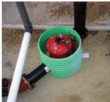
Workers added a 6-inch Netafim-ARAD Hydrometer hydraulically controlled pulse flowmeter before effluent heads to the dripfield.
