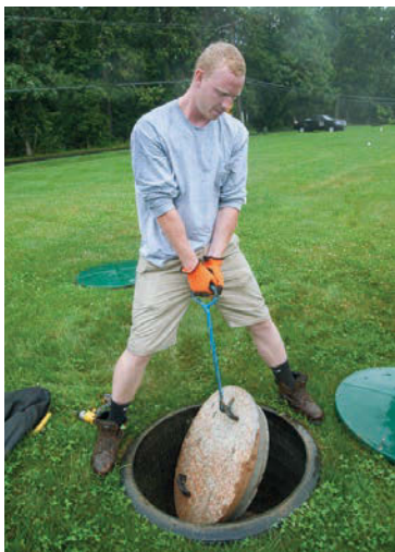
David Vincent pulls a septic tank lid in preparation for an inspection.
