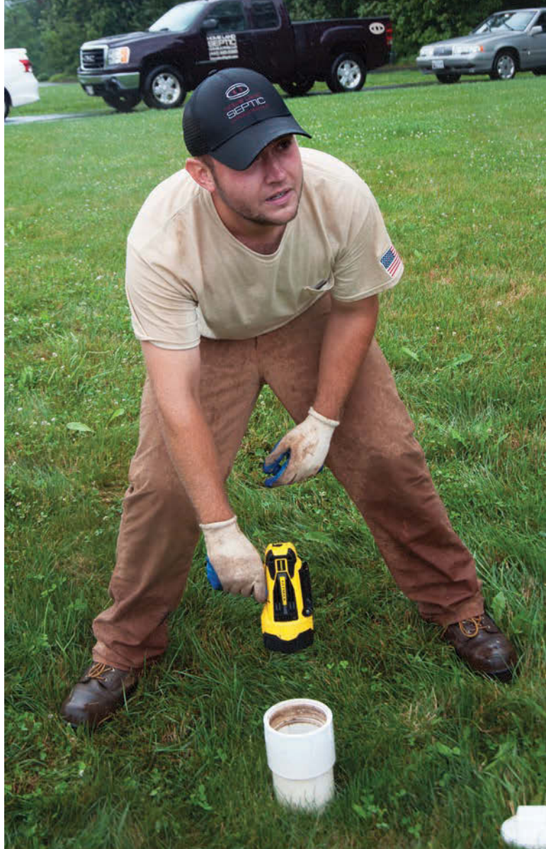
Dave Bancewicz inspects an observation port on a residential septic system.
