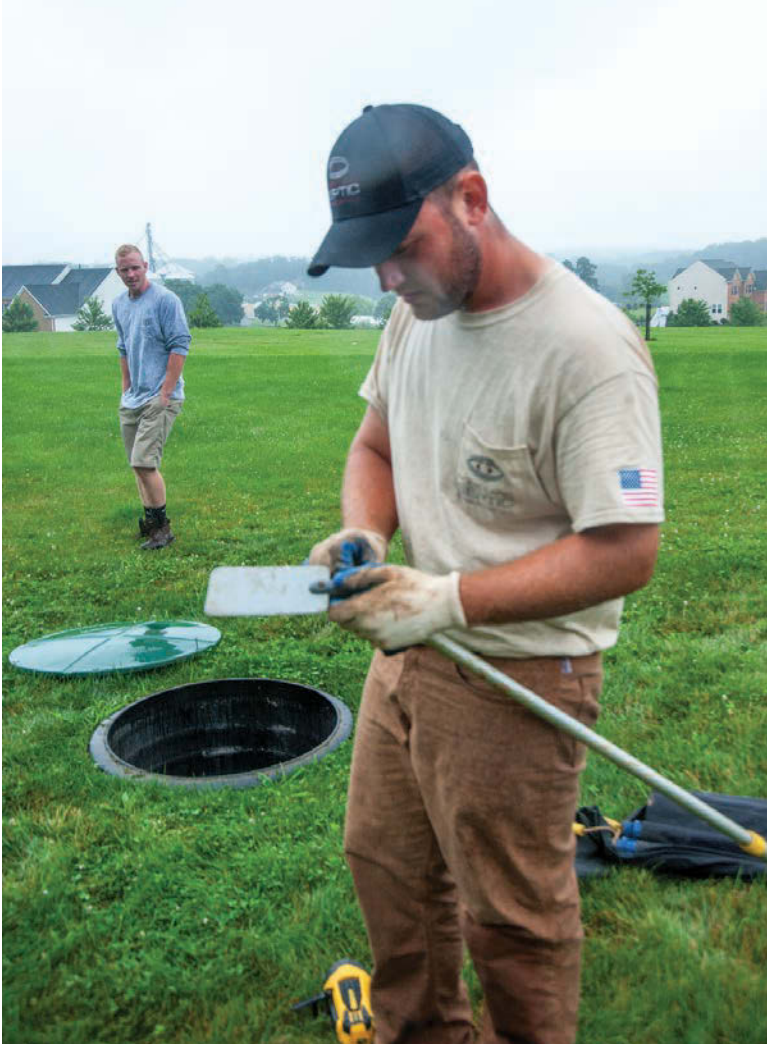
Dave Bancewicz assembles a pole and mirror to get a closer look inside a septic tank.
