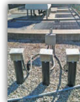
Elementary School, MO 3 Salcor 3G UV Units (Parallel Array) in Extended Aeration
