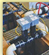
Nursing Home, OH 2 Salcor 3G UV Units in Series with an Activated Sludge Plant. Replaces Chlorination
