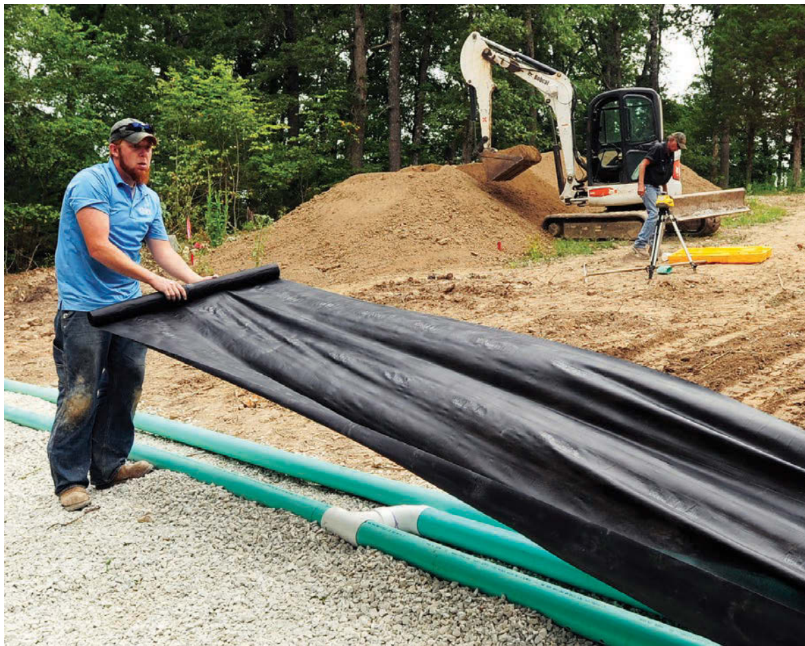
LEFT: All Clear Pumping & Sewer's Brent Kleffner lays down geotextile fabric over the pipes and aggregate absorption bed during an installation.
