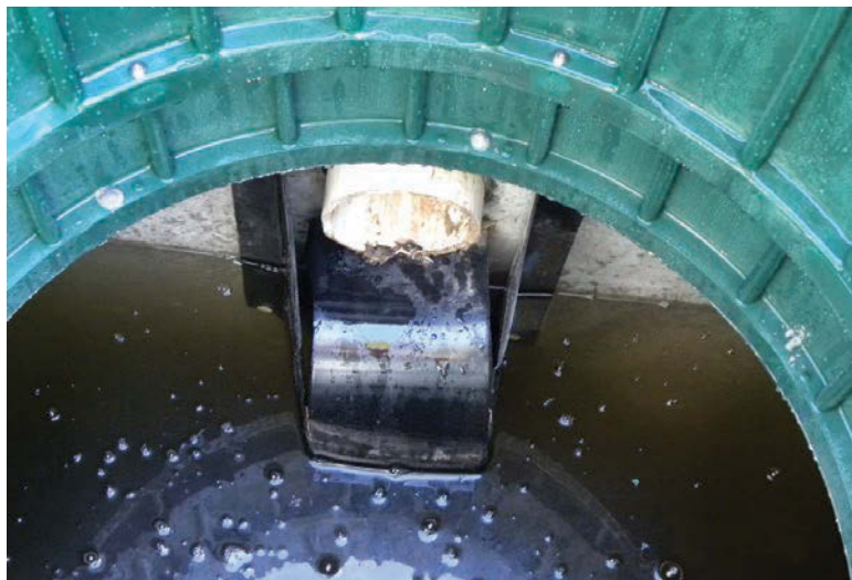
This image shows one service provider's solution to a plugged inlet. The configuration will not keep scum from blocking the inlet. (Photo courtesy of Jeff Burger)
