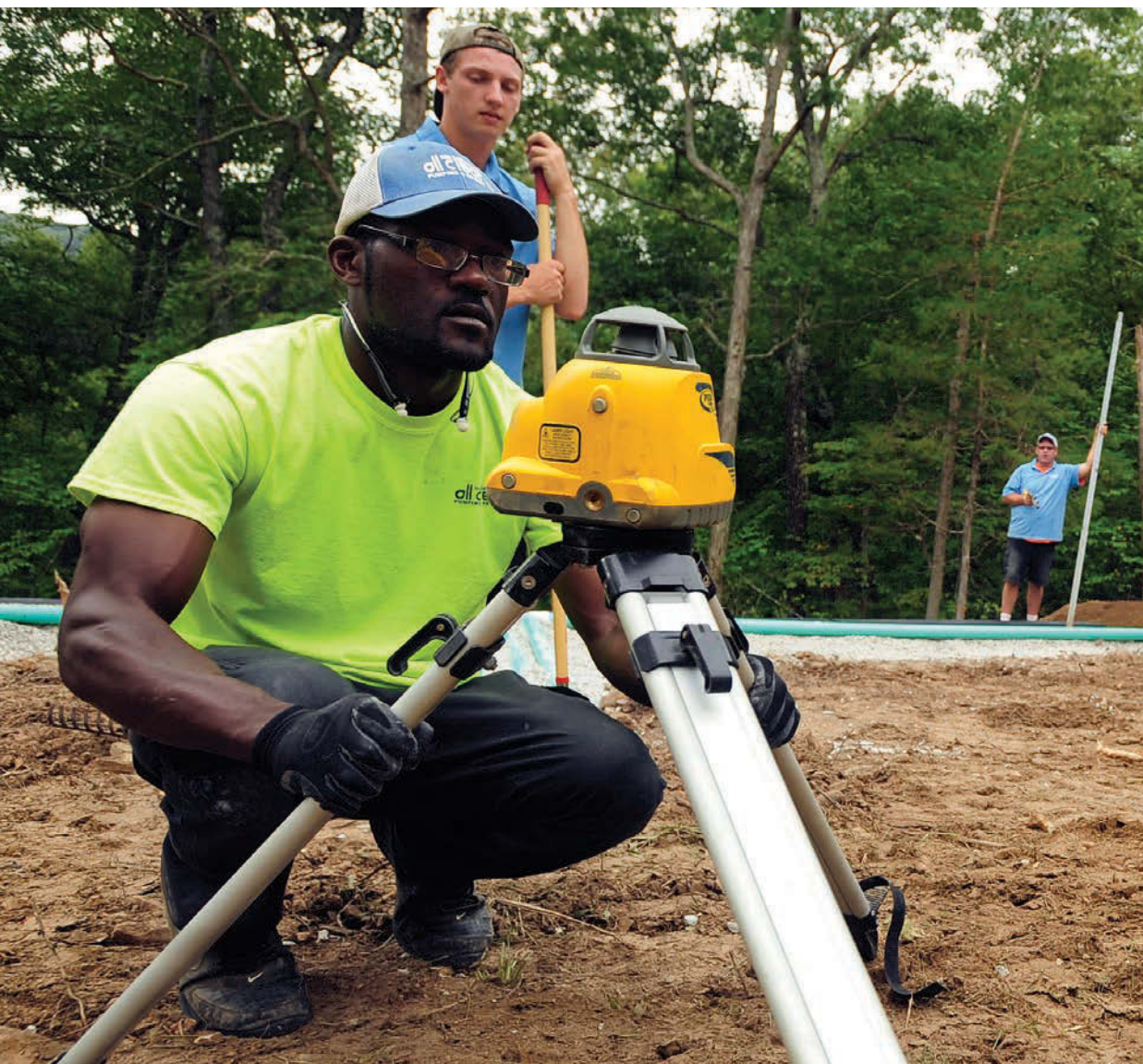
All Clear Pumping & Sewer's Kelvin Lee uses a Spectra LL300 laser level during a system installation in Fulton, Missouri.
