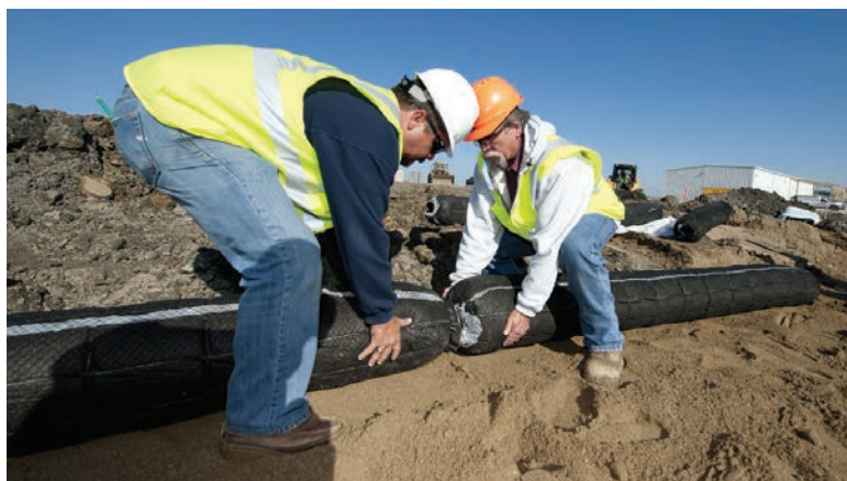
Zak Sherman from Infiltrator Water Technologies (left) and Mike Haddon from Indiana State Department of Health connect two conduits using the provided 4-inch internal pipe couplings. (Photos by Robert Densmore, Zen Photo Arts)
