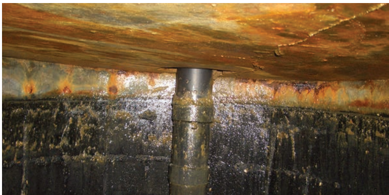
BELOW: A 1980s septic tank with inlet and outlet baffles precast through the lid. The T-baffle (not visible) is cast through the side. Note the closed outlet baffle and no signs of hydrogen sulfide deterioration. (Photos courtesy of Dawn Long)
