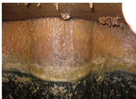
<<LEFT: A precast tank from 1979 with no air space above the baffles and no sign of hydrogen sulfide deterioration.
