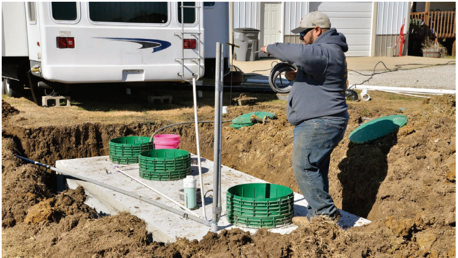
Jason Birdsong runs electrical lines during a system install. The risers and lids are from Tuf-Tite and the tank was provided by Allegiant Precast.
