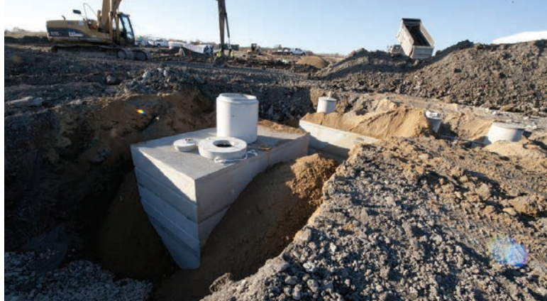
Backfilling continues around the two 3,500-gallon septic tanks and 3,500-gallon dose tank bedded on 24 inches of compacted crushed limestone.
