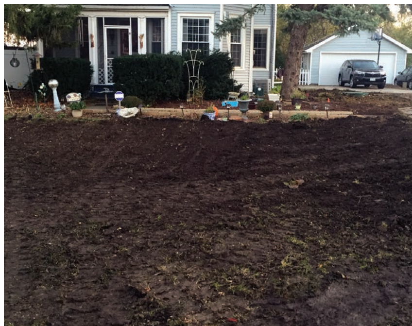
The completed MBR installation shows only a few riser lids peeping above grade. Notice the restricted space to the left and right of the home. The backyard was similarly small, necessitating placement of the drainfield in the front yard.
