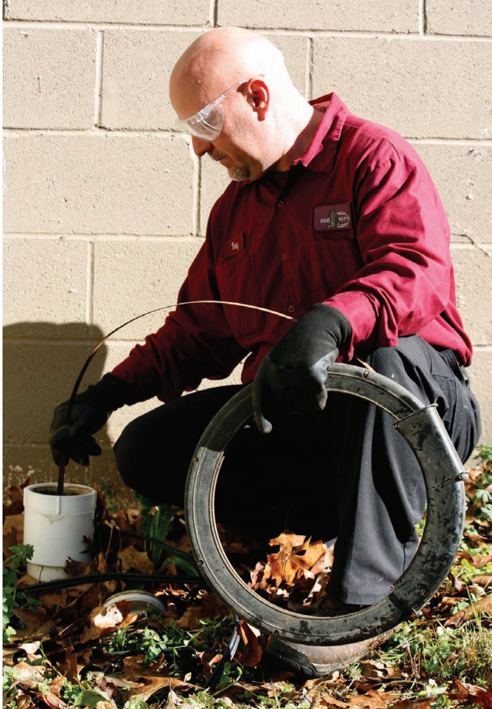
ABOVE: Tony Townsend runs a snake through a pipe to determine the distance between the house and a septic tank.
