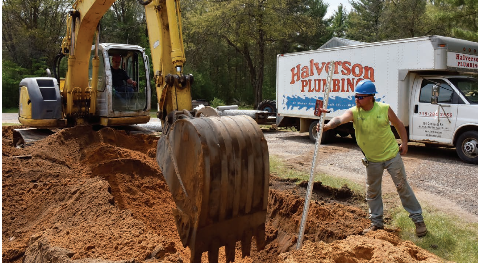
ABOVE: Dan Wiczorkowski measures trench depth as Jeff Stear works the Kobelco excavator while installing a new system for a one-bedroom apartment.
