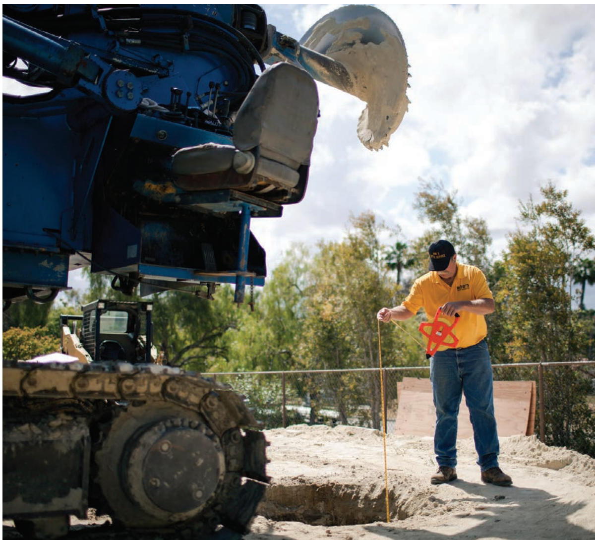
Willis confirms the depth of a vertical seepage pit bored by another contractor.
