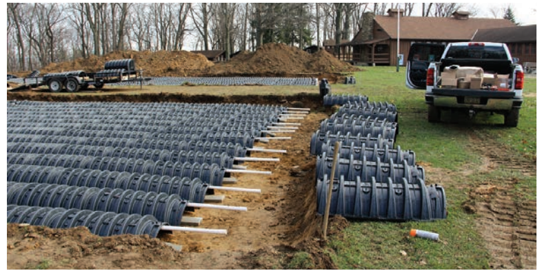
The 6,888-square-foot drainfield has two 42- by 82-foot zones, each with 28 laterals, 14 laterals per side for a total of 560 Quick4 standard chambers from Infiltrator Water Technologies.
