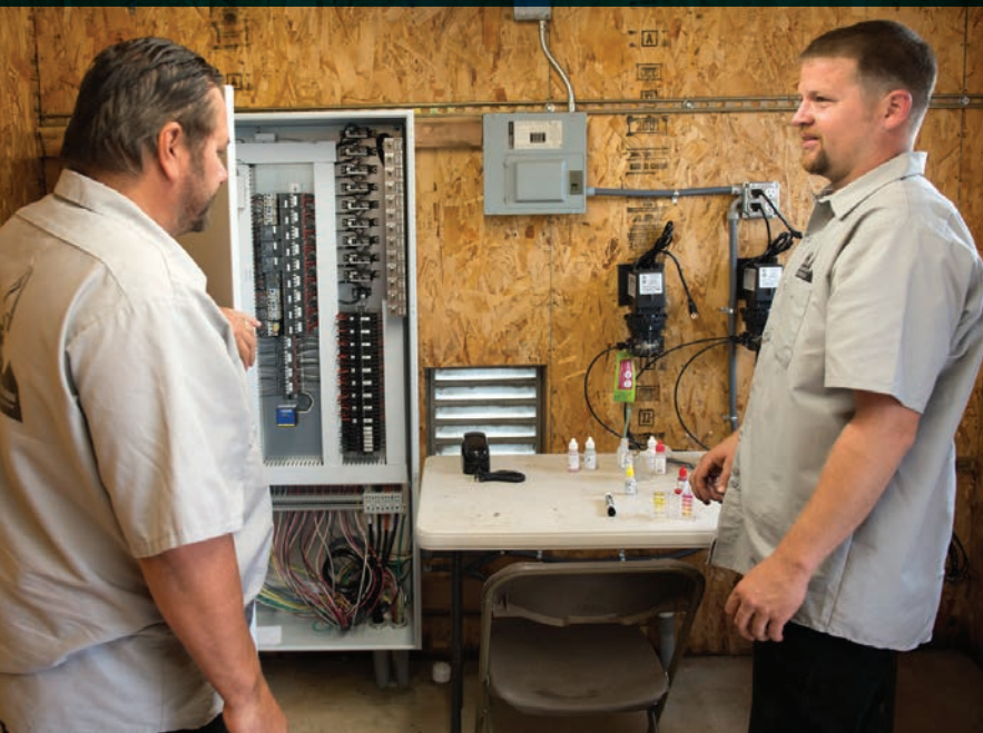
▼ Nick Herrera, left, and Nick Graham check the control panel for the Orenco AdvanTex AX-Max community treatment system installed by NH Construction.
