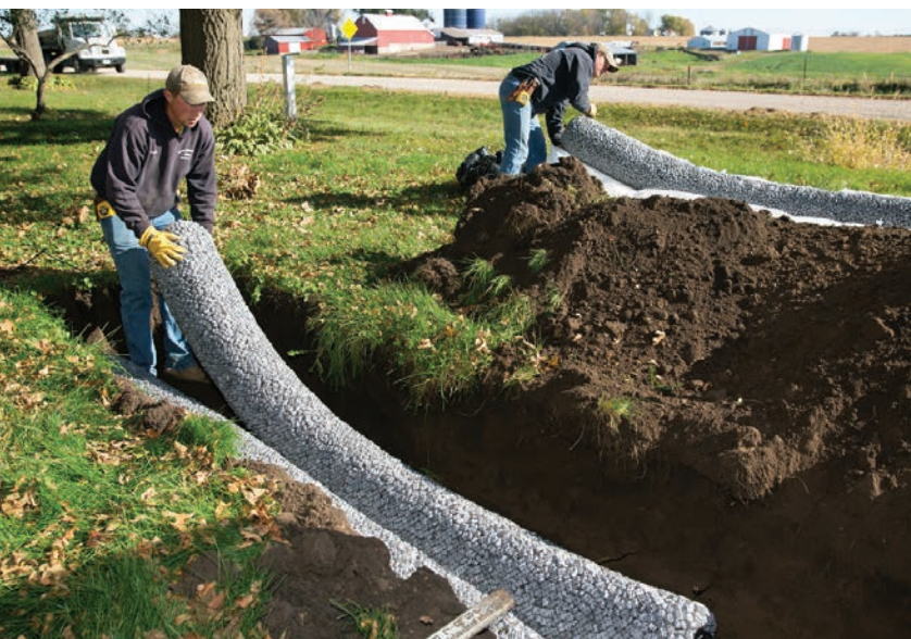
▲ Justin Rozendaal and Rick Beyer install EZflow bundles for a new drainfield system.
