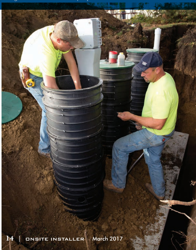
▼ Justin Rozendaal wires a Minuteman alarm post with two 20-amp circuits during an installation. The company uses Tuf-Tite lids and risers for tanks.
