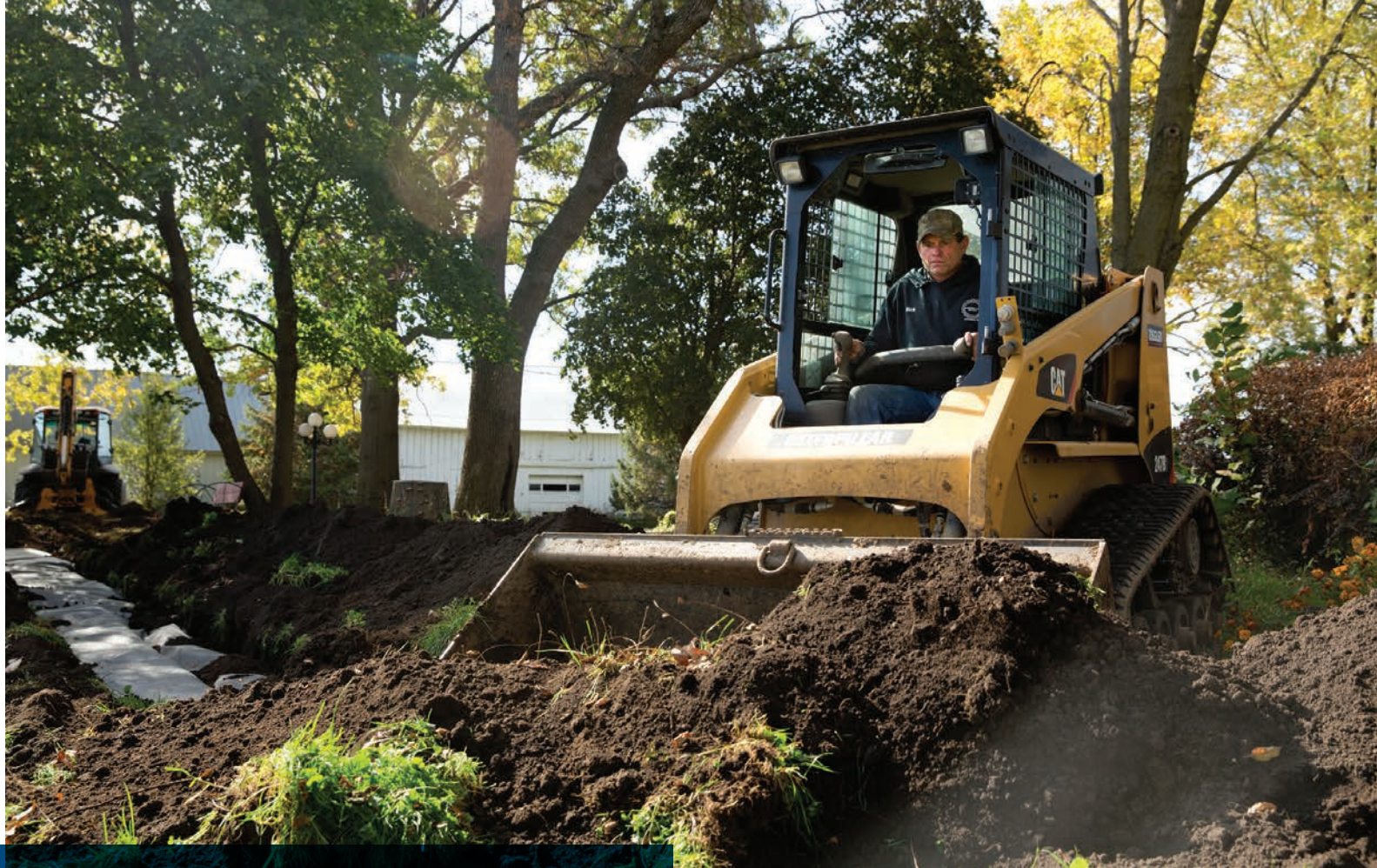
▲ Rick Beyer uses a Caterpillar 247B3 skid-loader to cover a drainfield.
