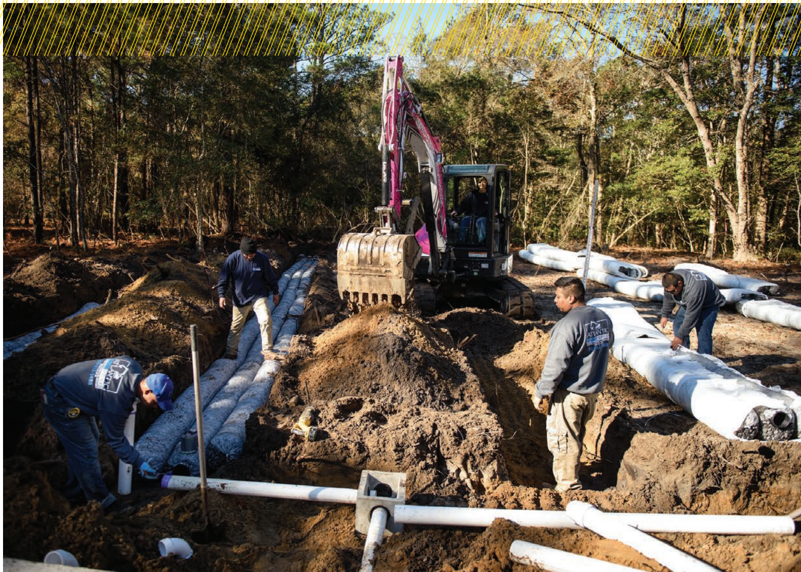
▲ The crew lays out a new drainfield using EZFlow media by Infiltrator Water Technologies, while Stephenson digs a trench.
