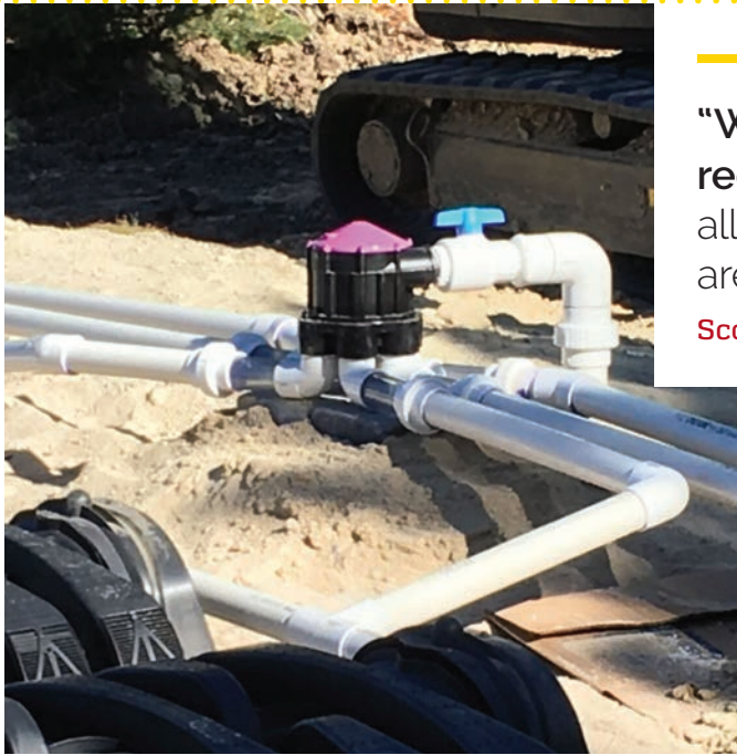
▲ The automatic distribution valve (Orenco) feeds six manifolds in the 102-by-36-foot sand filter.
