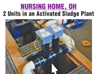
UL & cUL LISTED Test Proves 30-Day Underwater "FLOODPROOF" (NEMA 6P)
