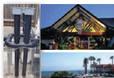
DUKE'S OCEANFRONT RESTAURANT, Malibu, CA 3G UV Units Parallel/Series Array Disinfects Effluent Discharging into Pacific Ocean Beach Sand
