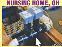
2 UV Unit Array Replaced Chlorine Chamber
