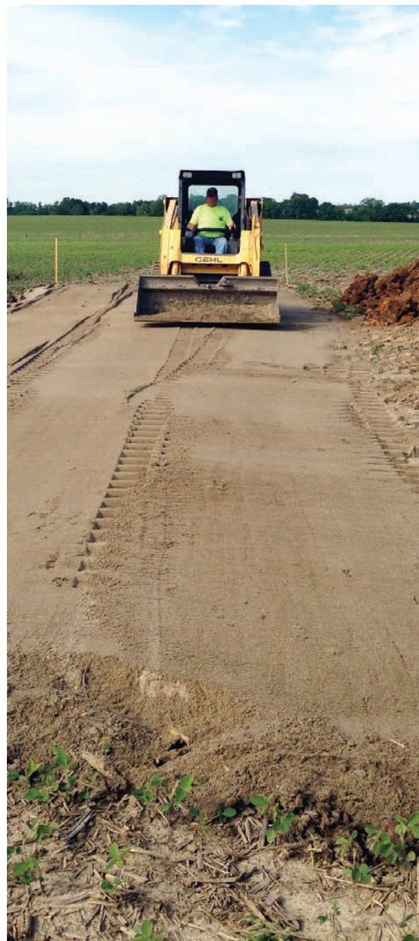
➤➤ Jeff Black levels sand over a new drainfield using a Mustang-Gehl CTL85 skid-steer. Dirt was brought in and mounded over the system.
