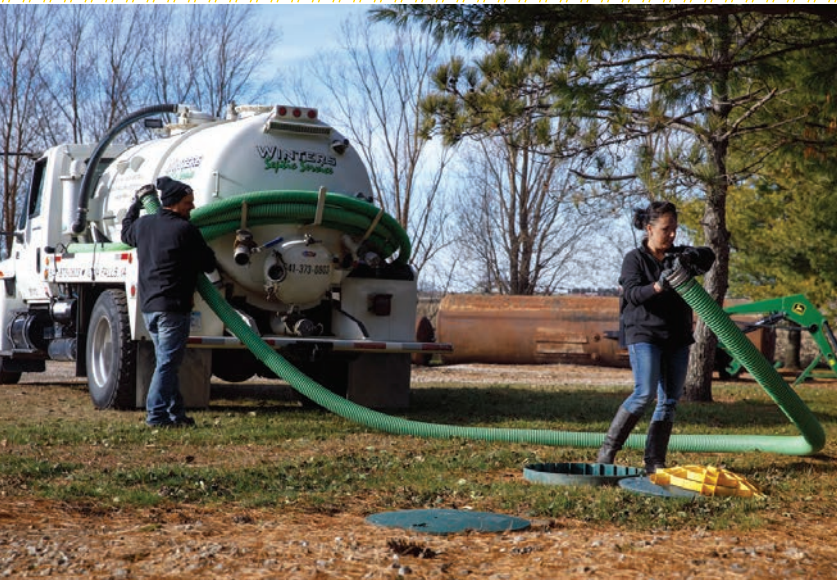
◀◀ Amanda and Trent Winters drag hoses to pump out a tank using their 2003 International 4300 vacuum truck with a Masport pump.
