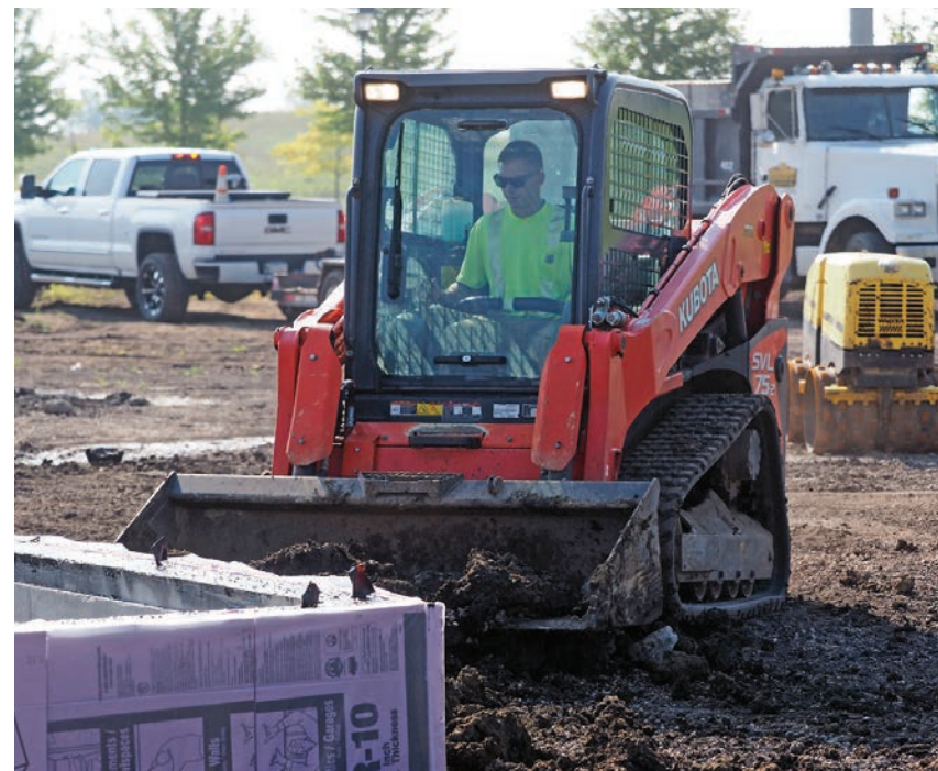
▲ Joshua Bruender operates a Kubota track loader on a job site.
