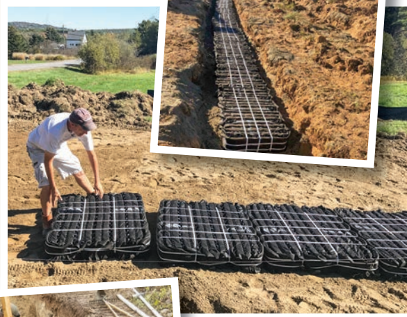
Habitat for Humanity, Maine
