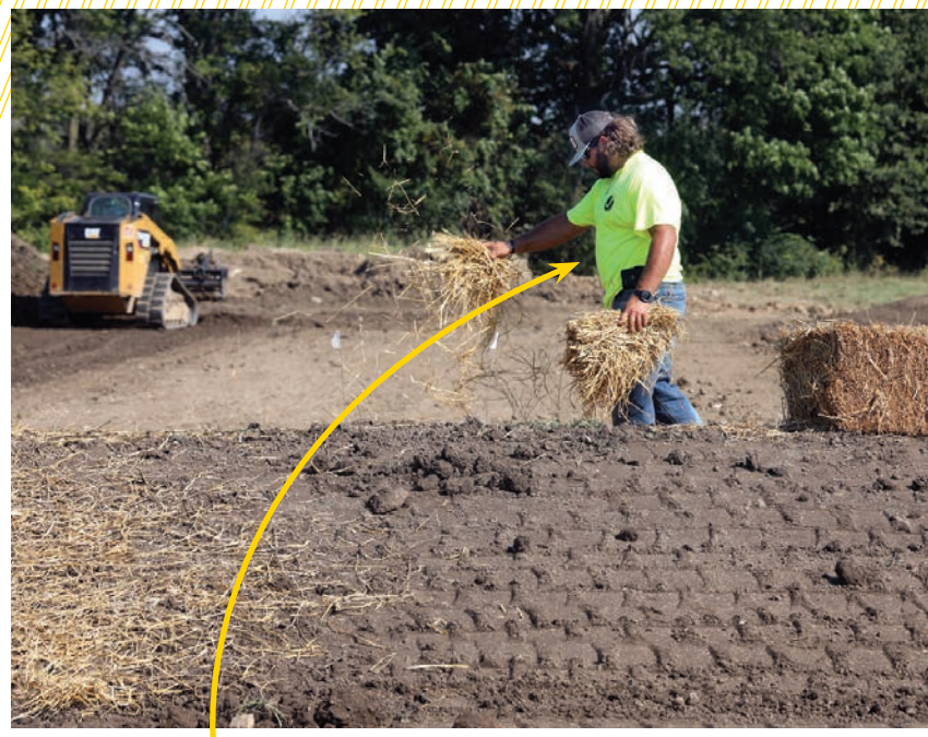
▲ Technician Austin Garcia spreads hay over a mound after seeding for ground cover.
