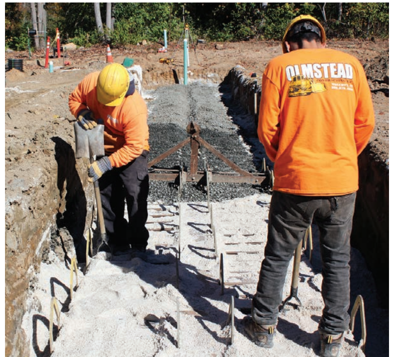
▲ Jose Vazquez (left) and Alfred Brown from Olmstead Contracting compact C-33 sand with the D-grip handles on their shovels.
