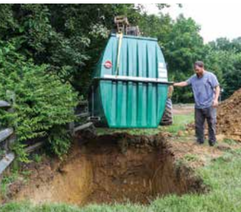
▲ Ray Harrison guides the AdvanTex AX20RT from Orenco Systems into its resting spot.
