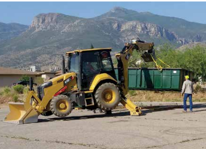
◀◀ Foreman Zak Long of American Septic Service uses a Caterpillar 461F2 backhoe loader to unload a 2,000-pound AdvanTex AX100 module (Orenco Systems).
