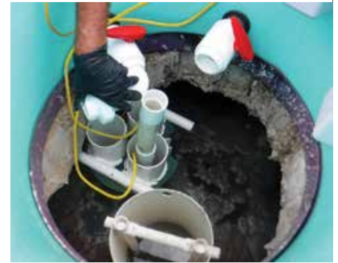
▲ Foreman Zak Long of American Septic Service and Jared Struse, owner of Sierra Vista Plumbing, assemble plumbing for the recirculating valve and Biotube pump package (Orenco Systems). Both wear Chill Pad cooling towels to work in temperatures above 100 degrees F.
