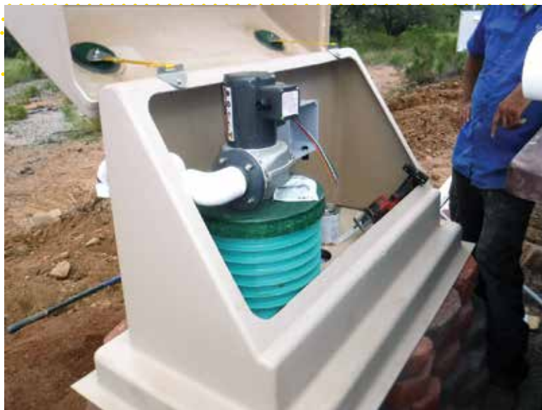
▲ The vent fan assembly for the AdvanTex AX100 modules (Orenco Systems).
