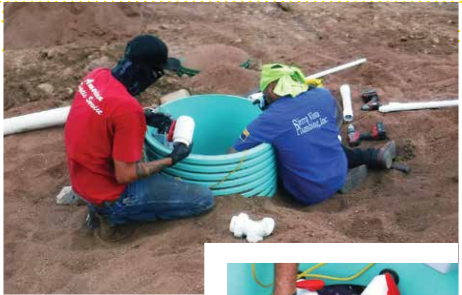
▲ Foreman Zak Long of American Septic Service and Jared Struse, owner of Sierra Vista Plumbing, assemble plumbing for the recirculating valve and Biotube pump package (Orenco Systems). Both wear Chill Pad cooling towels to work in temperatures above 100 degrees F.
