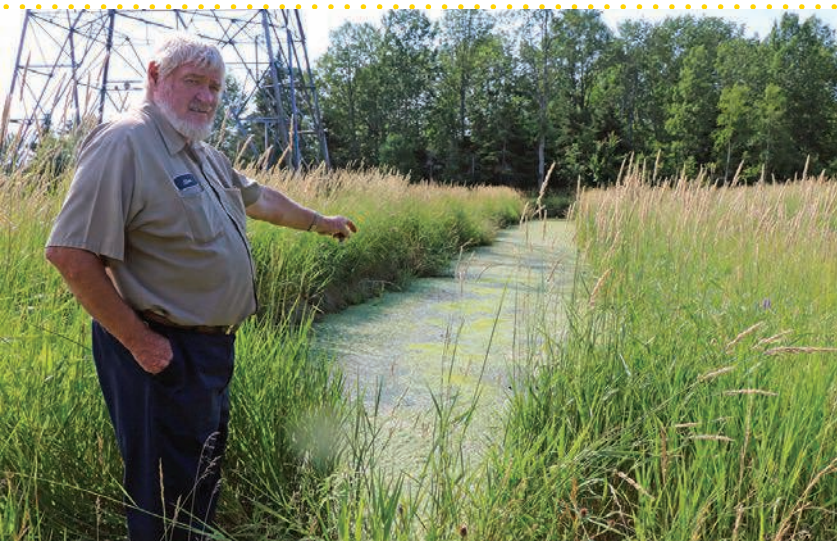
◀ Allan Baird, owner of Baird's Septic Tank Pumping, looks over the company's settling lagoon where cattails filter wastewater. (Photos courtesy of James Baxter)
