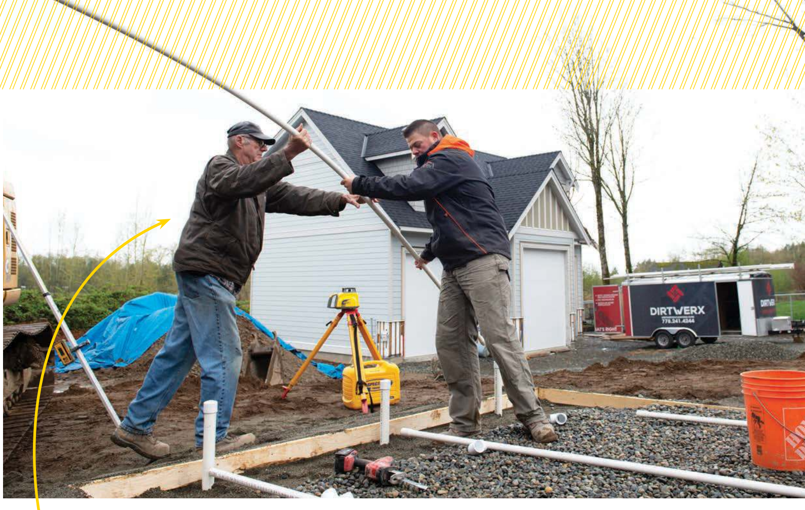
▲ Tim Wilson, left, and Clint Watrich install PVC pipes for a residential onsite system. A Spectra Precision GL412N laser level is shown in the background.
