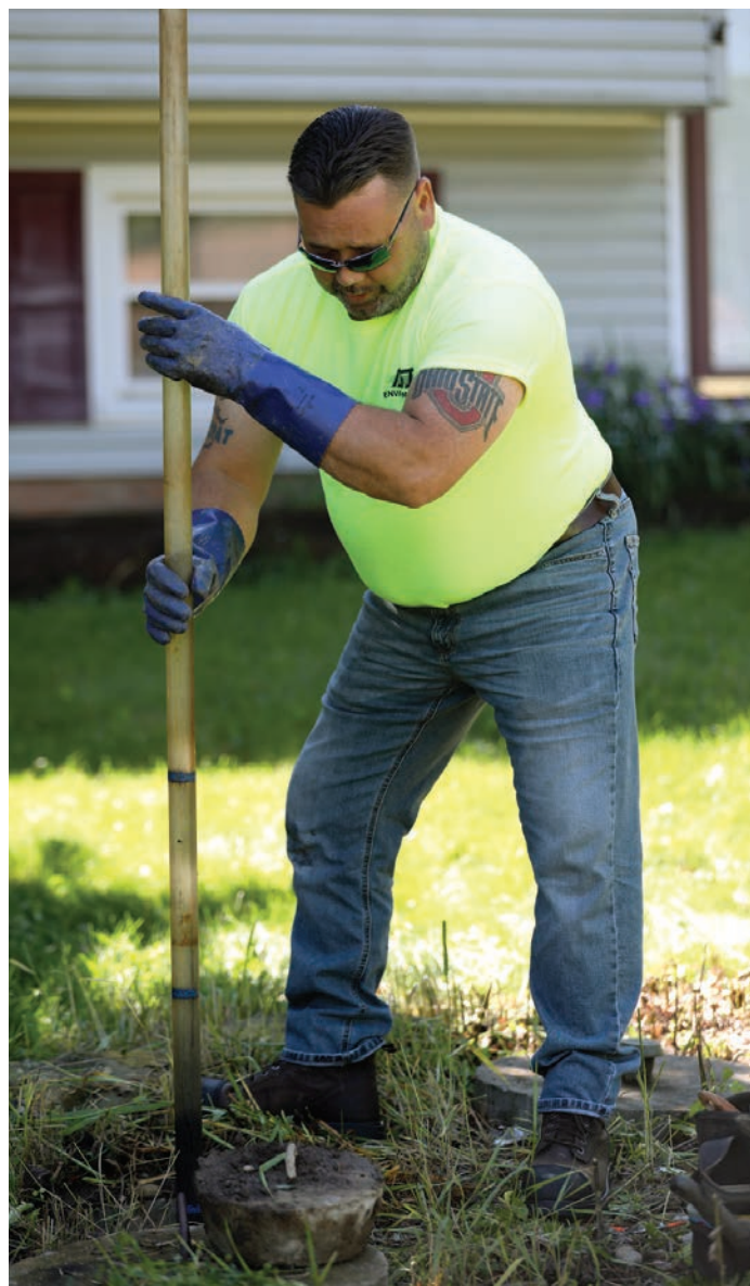
▲ Technician Ken Saltz uses a Sludge Judge (Nasco Whirl-Pak) to measure solids in a residential tank during an onsite maintenance call.
