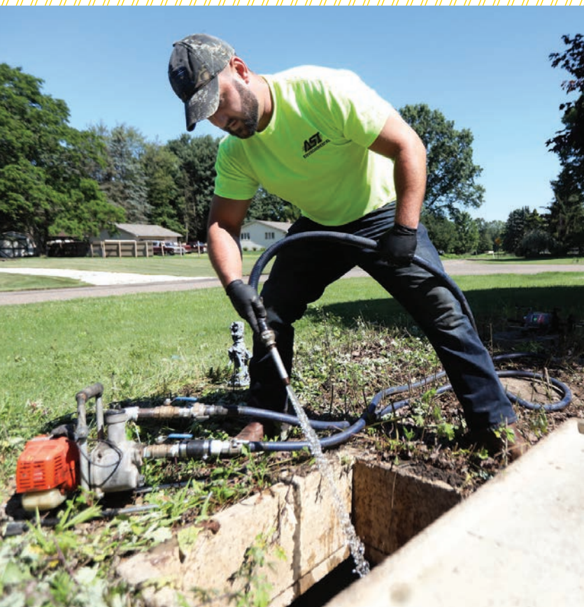
▲ Ryan Wallace uses an Echo WP1000 fluid pump to clean an upflow filter.
