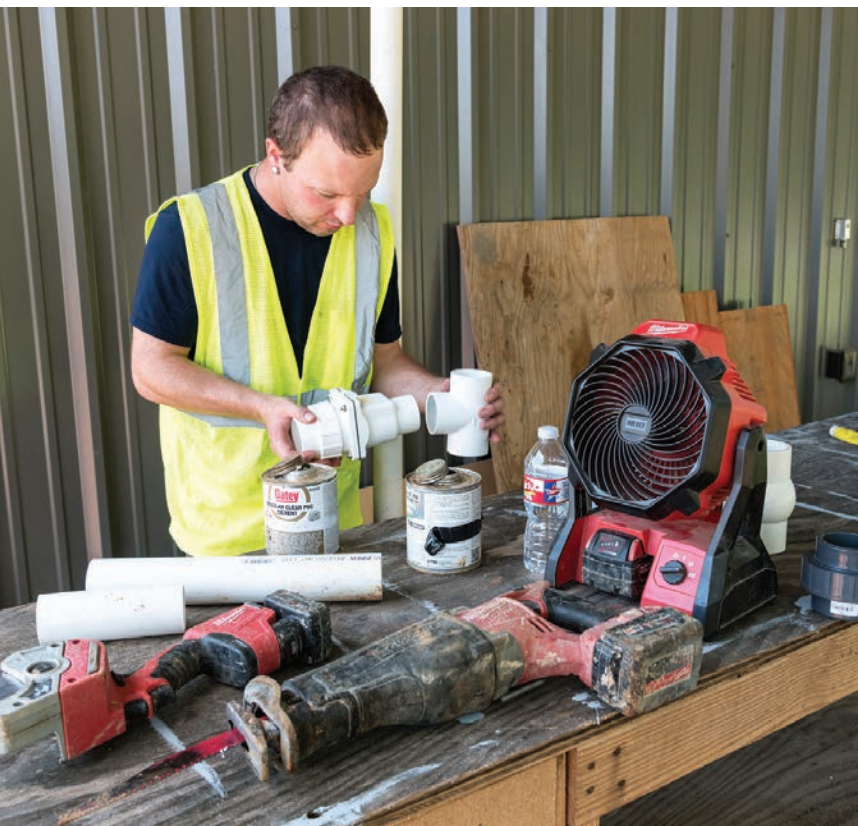
▼ Technician Adam Ault at the workbench, piecing together PVC connections for a new onsite system in Little Rock, Arkansas.
