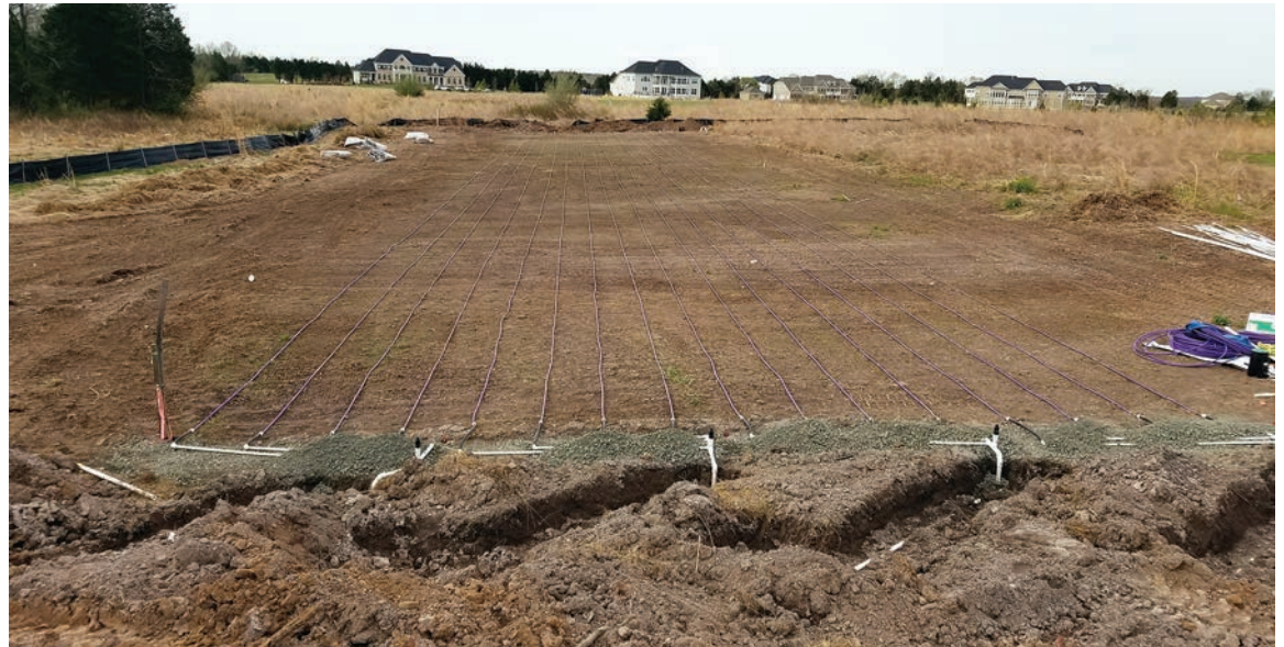
▼ Installation of a drip field for a single-family home.
