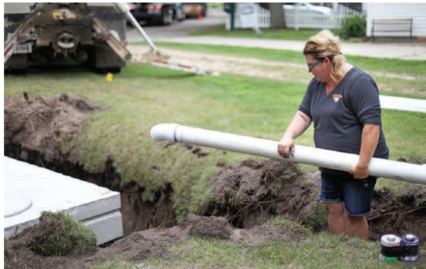
▼ Becky Richards runs PVC pipe to a new septic tank for a residential system.
