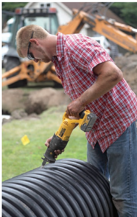
▲ Zach Rodriguez cuts corrugated pipe from Advanced Drainage Systems.
