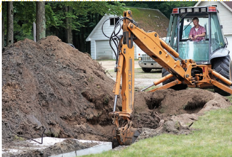
▲ Zach Rodriguez uses a Case backhoe to dig a trench leading to a new septic tank.
