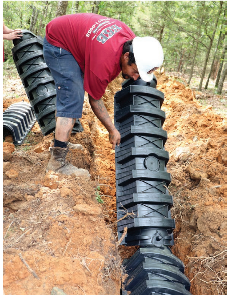
▼ Technician Mummert lays Infiltrator Water Technologies Quick4 Equalizer 24 chambers at the site of a system replacement project in Fayetteville, Arkansas.
