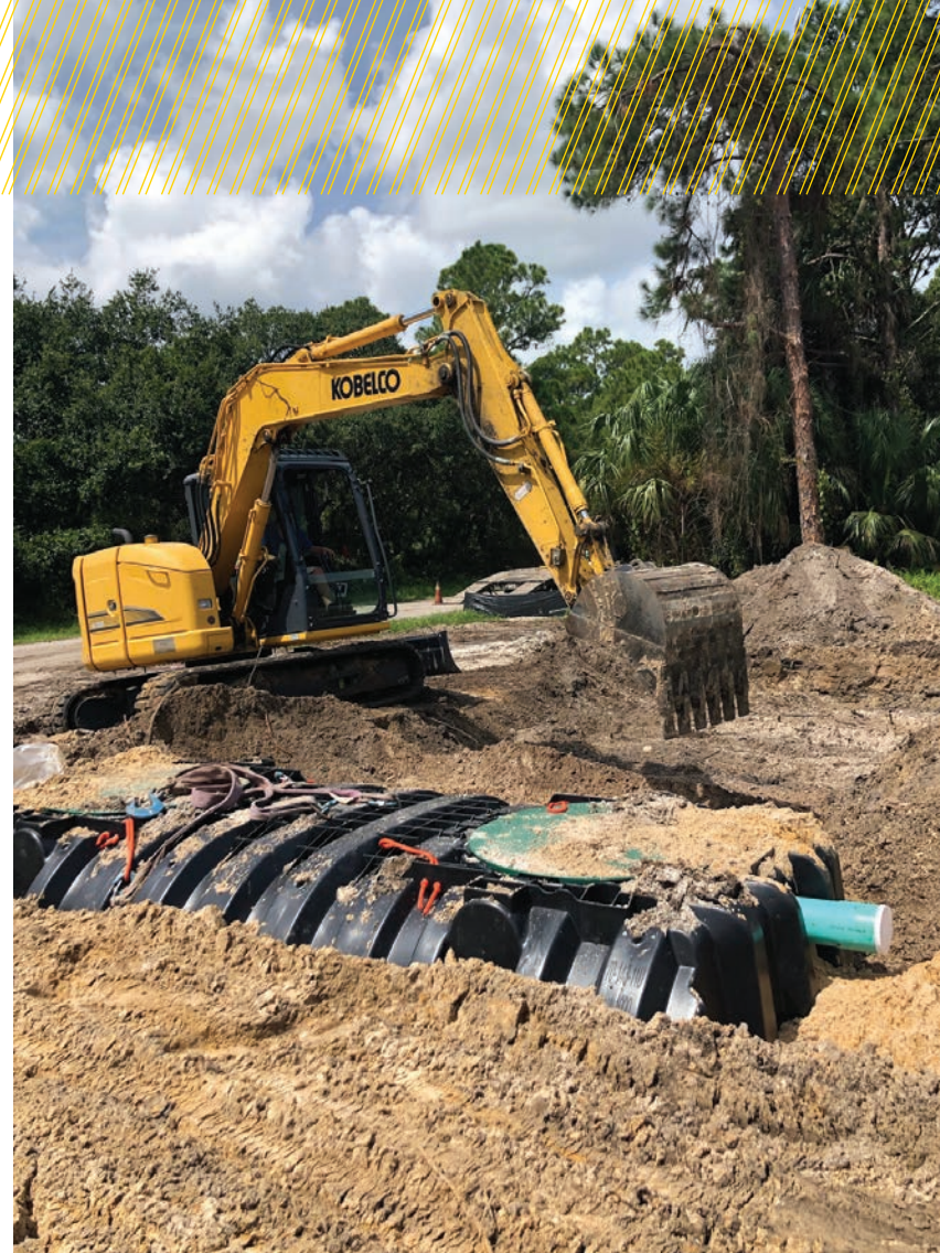
▲ Zach Grantham uses a Kobelco excavator to create a drainfield bed. The project featured products from Infiltrator Water Technologies.
