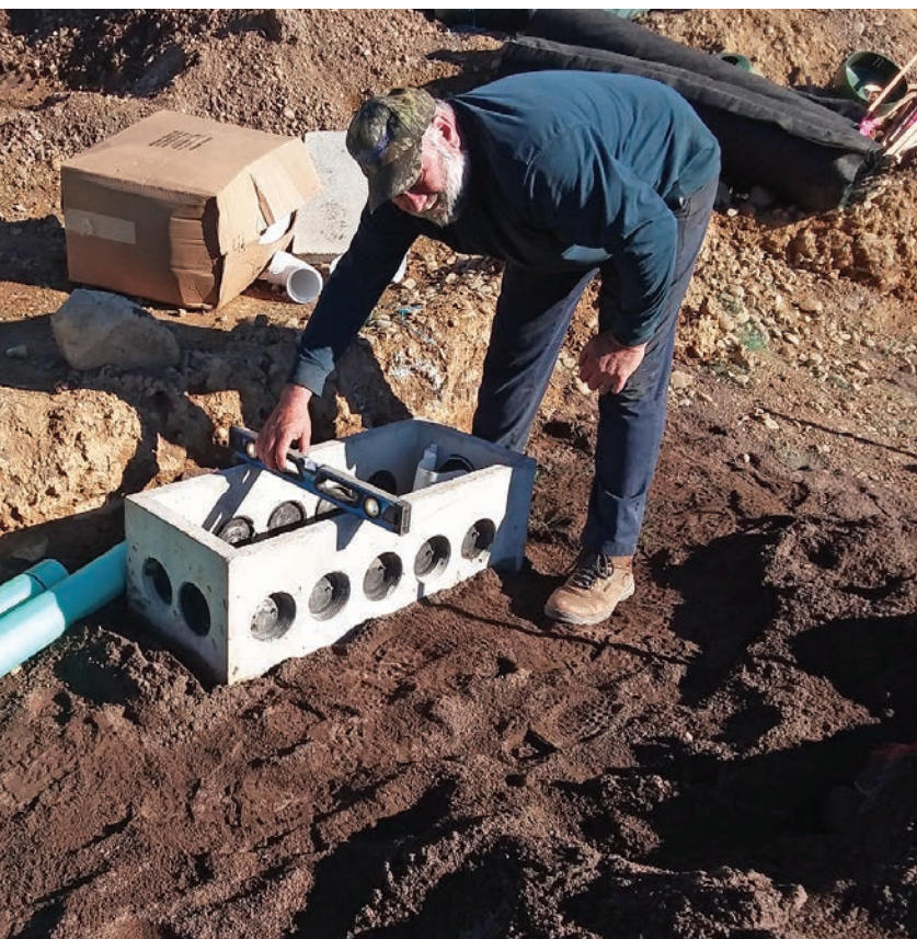
◀ Gary Royce Jr., owner of A+ Excavating, checks the level of a distribution box.
