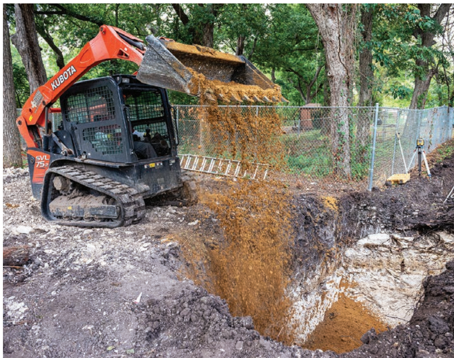
▼ Willard Cavitt operates a Kubota skid-steer, adding sand to the bottom of a trench.
