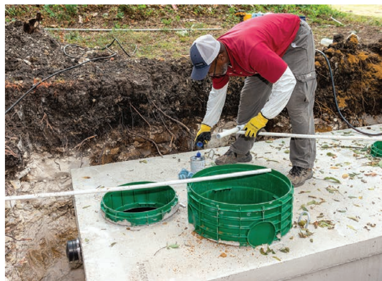
▲ Willard Cavitt runs PVC tube to a tank during installation. Risers and lids are from TUF-TITE.
