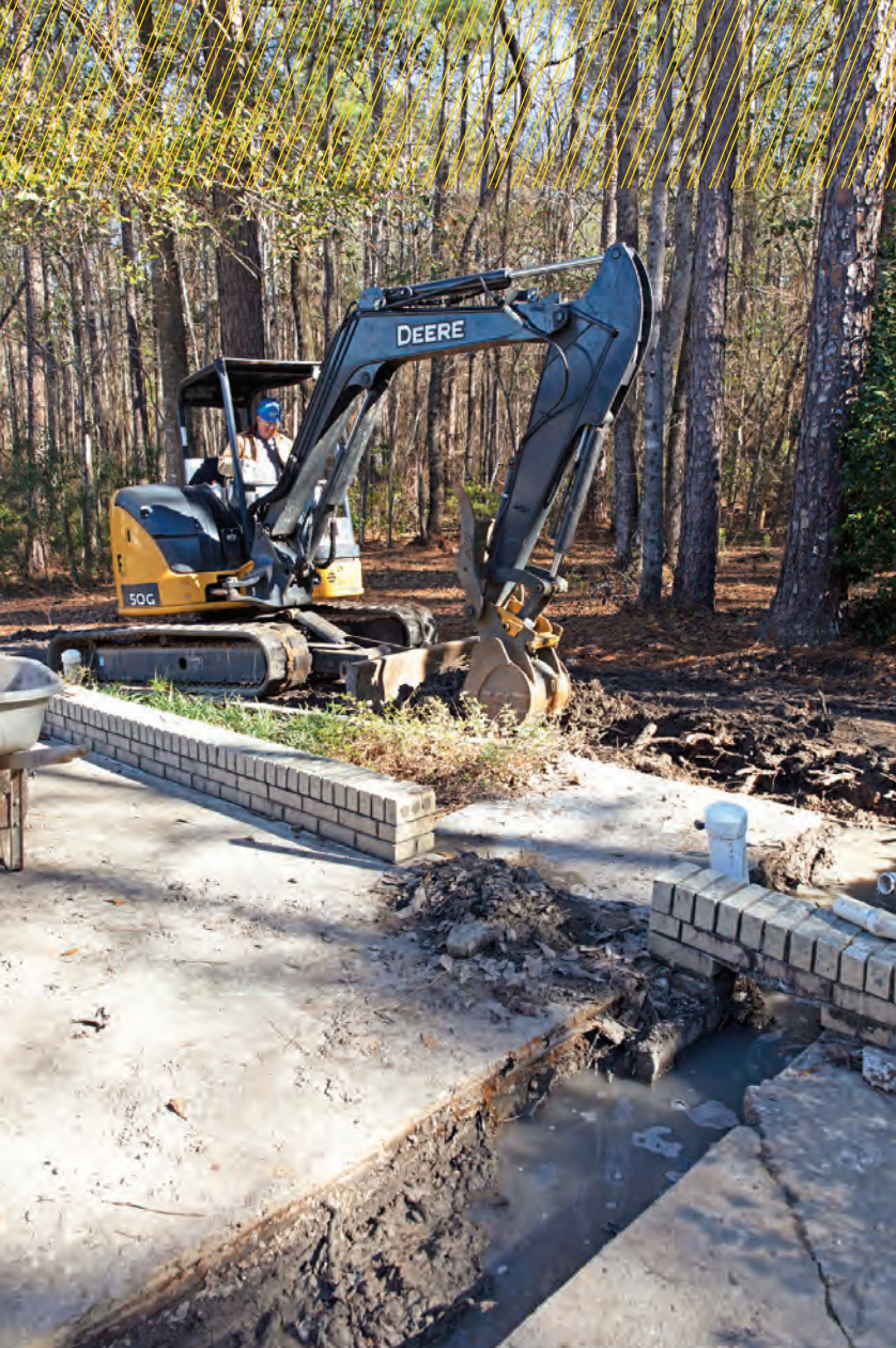
◀◀ Barney Allen digs a trench with a John Deere excavator.
