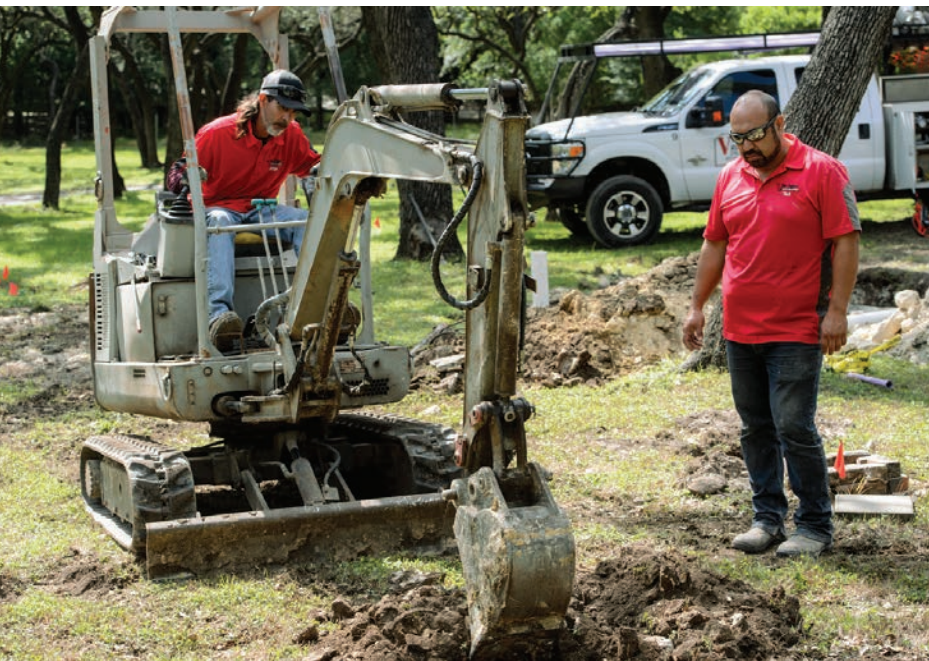
▲ Jorge Garza operates a Takeuchi mini-excavator at a work site.
