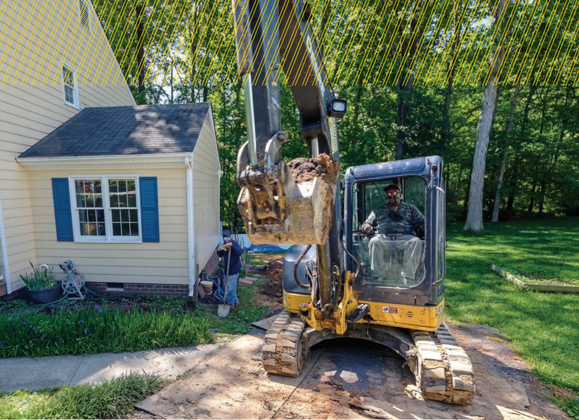
◀◀ The Stamie E. Lyttle Co. crew works on a residential system.
