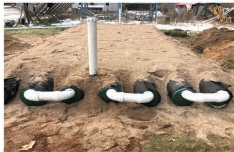
First AFS installation in Wisconsin, November 2019.
