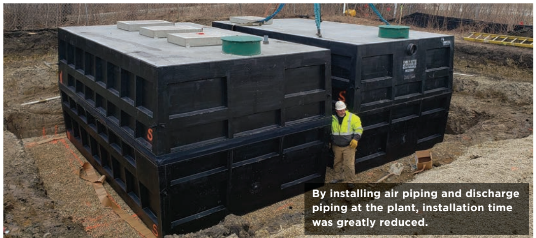
Workers install 12,000-gallon precast concrete tanks for a development in the Midwest.
