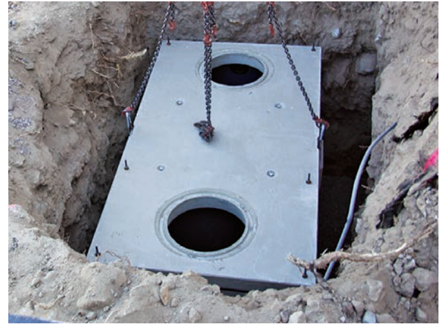
Photos courtesy of Jensen Precast
