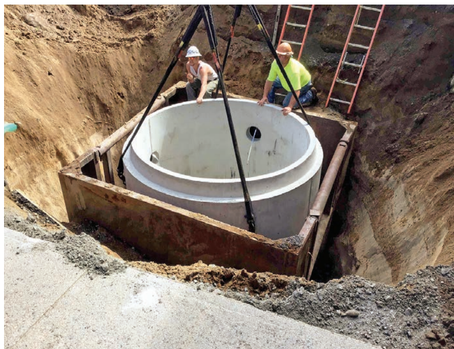
▼ Danny Stone (left) and Barry Cook from TJ Fiacco Construction help guide a riser onto the manhole base.
