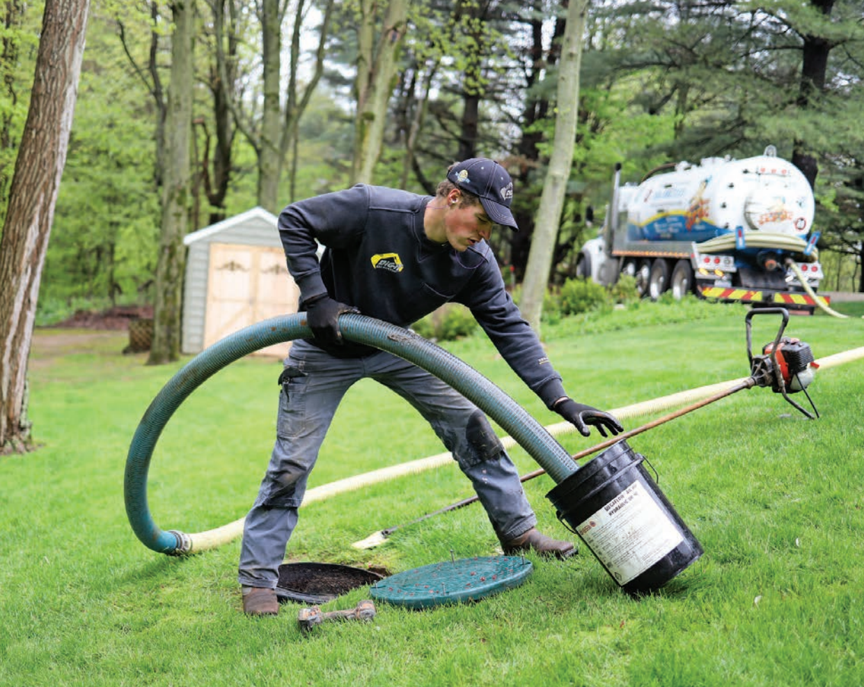
▲ Joshua Sanders rinses hoses after pumping a septic tank. Shown in the photos is a Crust Buster tank agitator and Kenworth truck built by Curry Supply and carrying a National Vacuum Equipment blower.
