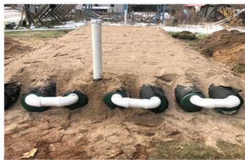
First AFS installation in Wisconsin, November 2019.
