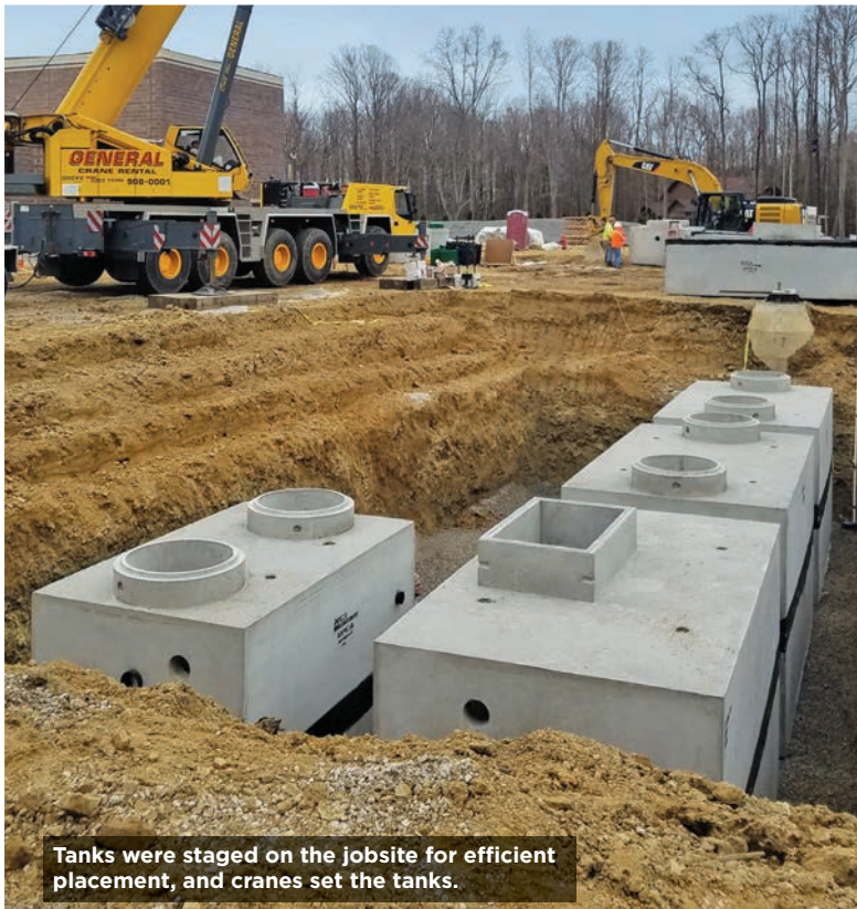
The 3,000- and 5,000-gallon tanks were 6-by-10 feet and 7-foot-6-inches-by-14-feet in size.
