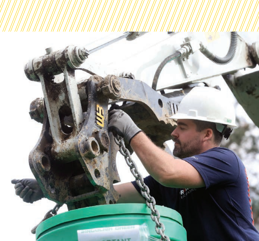
▲ Joe Bruening, of Bruening Excavating, works with a Norweco Singulair system in the field.
