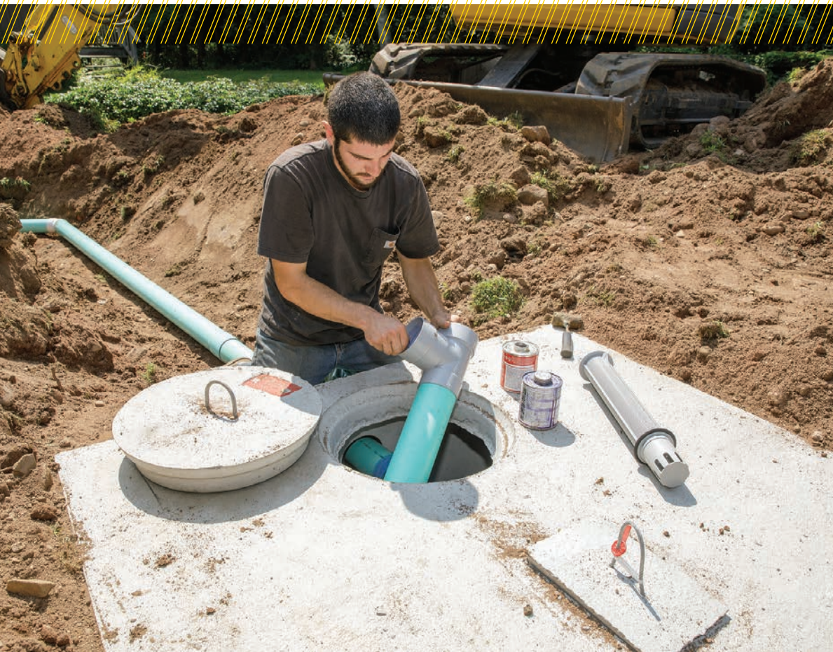
▲ Camarota installs an outlet baffle in a concrete septic tank.
