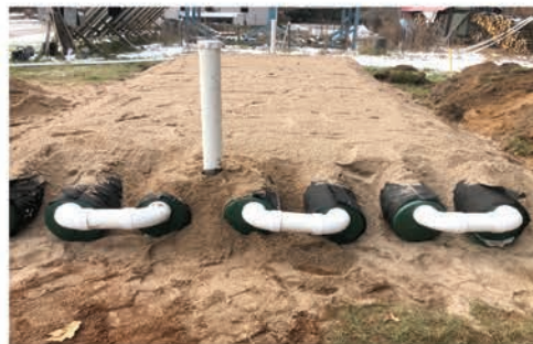
First AFS installation in Wisconsin, November 2019.
