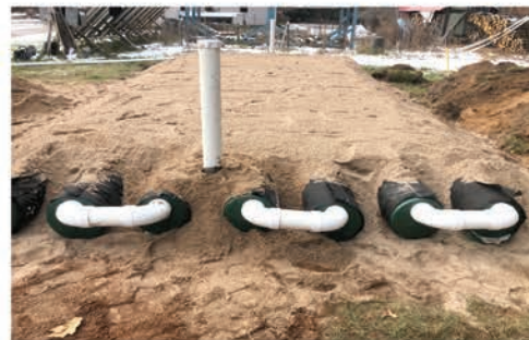
First AFS installation in Wisconsin, November 2019.
