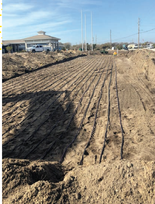
▲ Dispersal of treated wastewater is in a dripfield in front of the main Coral Bay Club building, visible at left. The field was covered and seeded and became a large lawn.
