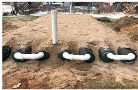
First AFS installation in Wisconsin, November 2019.
