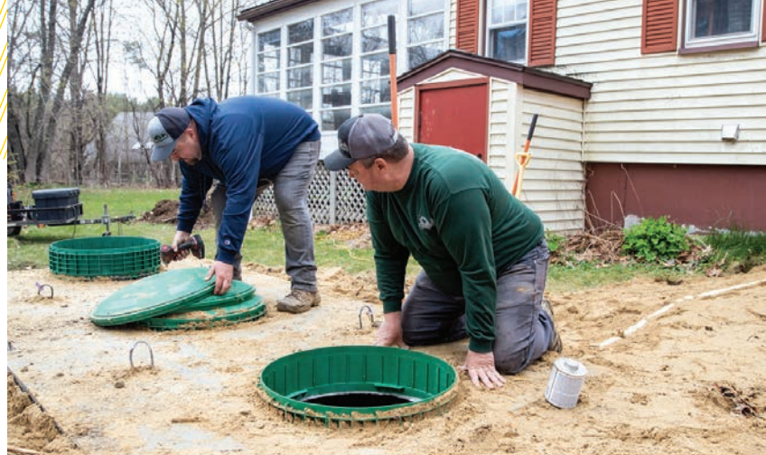
» Luke Rotti, left, and Earl Baxter organize the lids for Tuf-Tite risers being installed in a new septic system.
