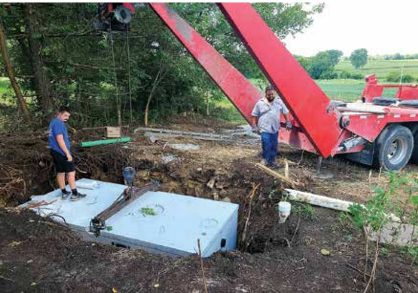
◀◀ Clint and Bryson McCammon installing an Allied Concrete Products tank.
