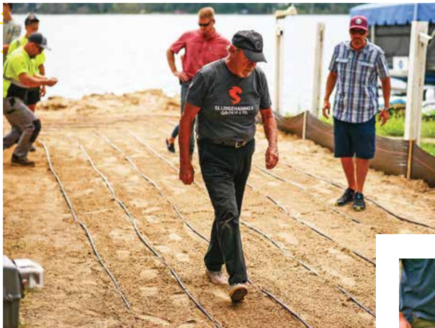
◀ Dan Wickham, center, inventor of SludgeHammer, walks the dripfield during the educational outing for the Paw Paw job.
