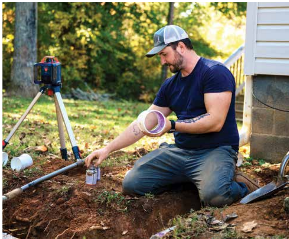
▼ McLaughlin prepares new pipe running from the house to a new septic tank the crew just installed.
