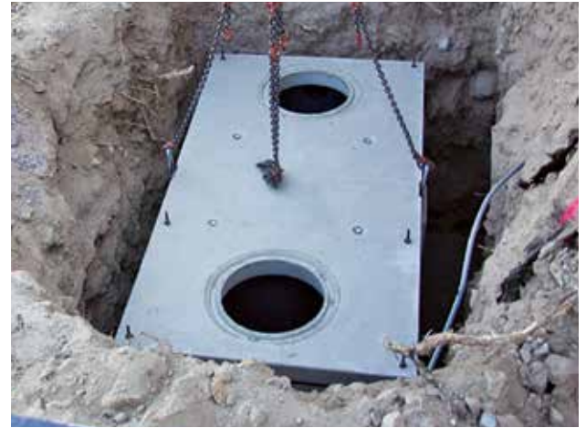
Photos courtesy of Jensen Precast
