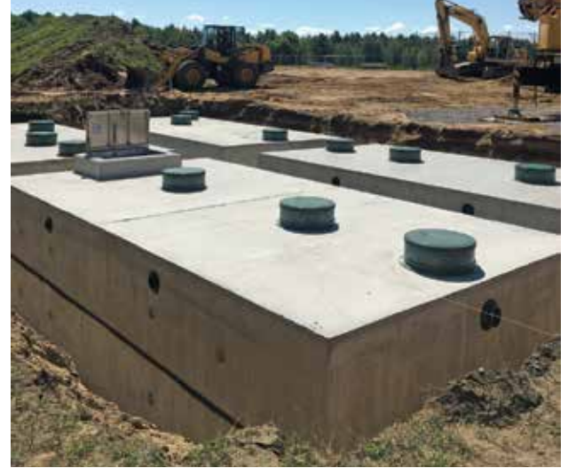
Photos courtesy of Camp Precast Concrete Products Inc.
